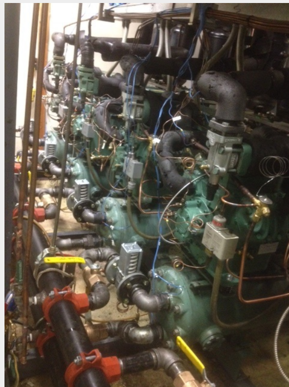
Photo by MSC: complex inner workings of a pharmaceutical lyophilizer taken during full system overhaul including refrigerant conversion
